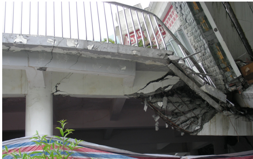
Figure 2. Typical example of the beam shear failure caused by the impact loading from the collapsed adjacent building (source: http://nees-anchor.ceas.uwm.edu/ ).
