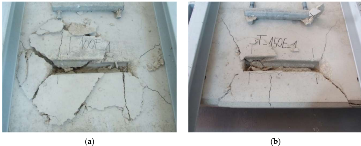
Figure 4.13 Breakout patterns: (a) in-field installation – h = 100 mm; (b) installation near the edge – c_1 = 150 mm
