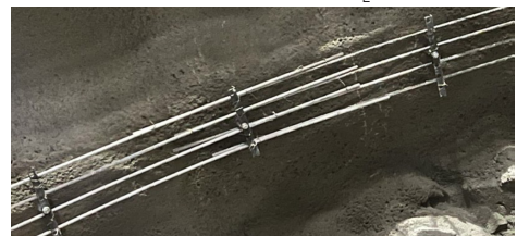
Figure 2 The arrangement of the bars before application of the covering layer of sprayed concrete. T-pieces used to create an arch
