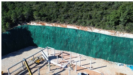
Figure 4 Finished part of the protected slope
