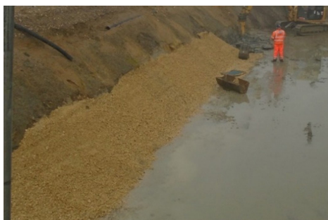
Figure 7 Construction of Angular Drainage Stone Key
