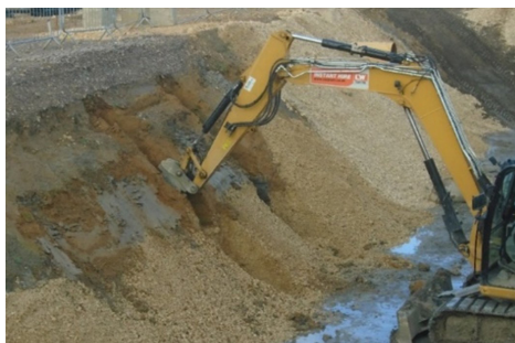
Figure 8 Construction of Cemented Aggregate Columns
