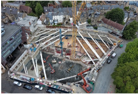
Figure 1 Basement Excavation and Propping
